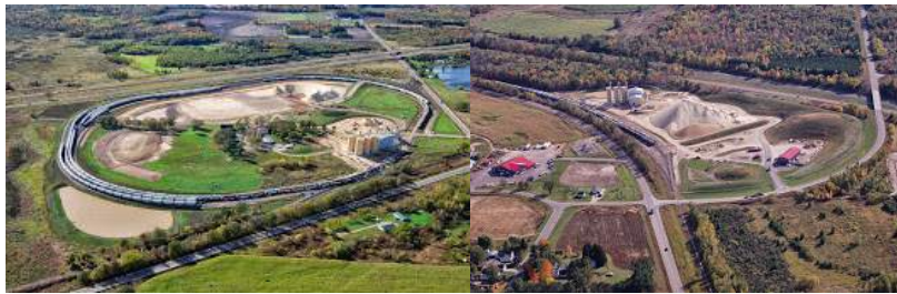
Figure 10. Typical impacts to road and infrastructure from frac sand mining (Photos by Ted Auch).
